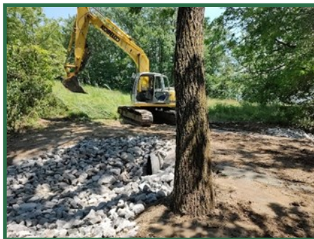
New culvert and stream crossing during construction.
